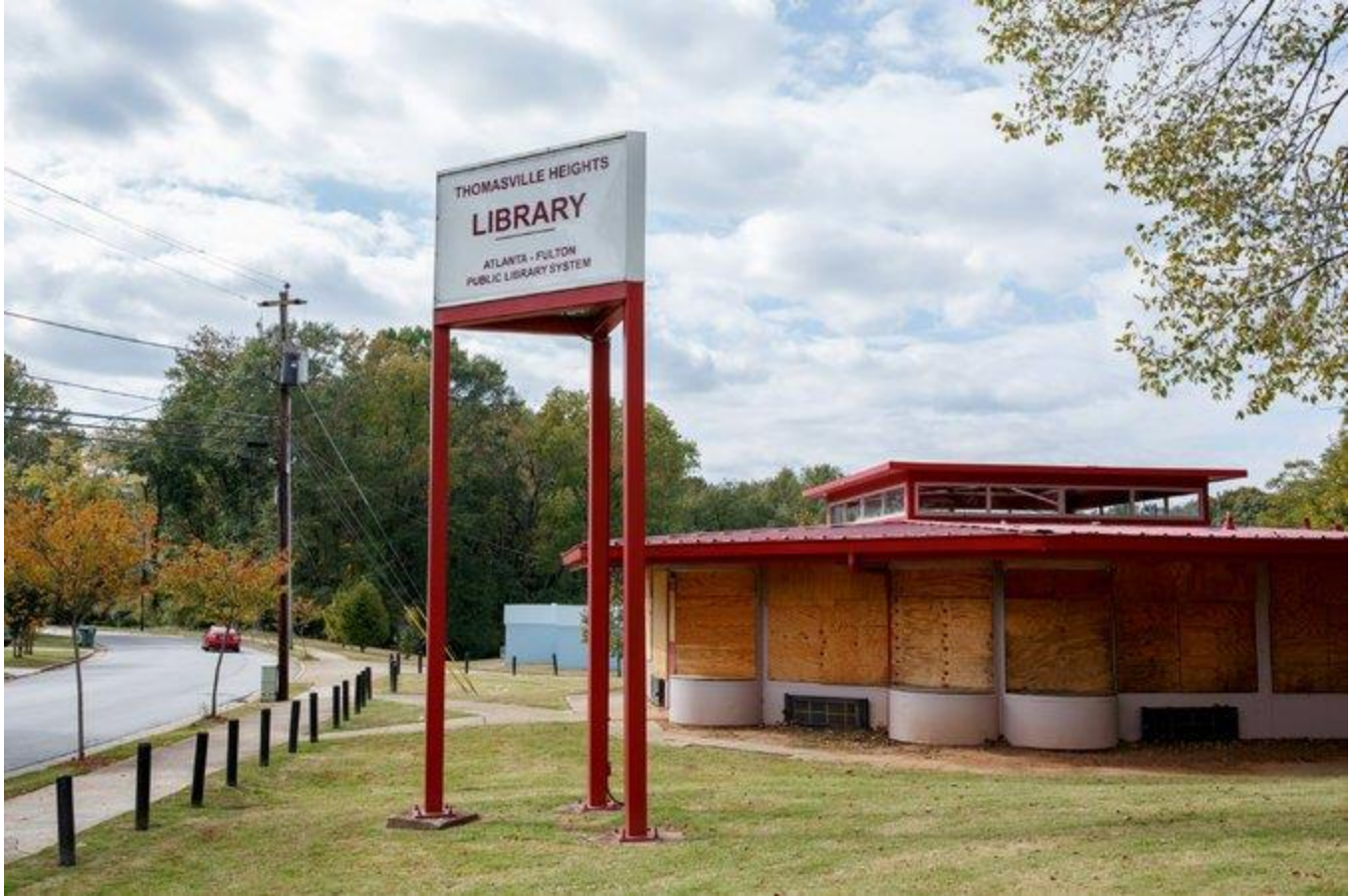
The library in the Thomasville Heights neighborhood is closed and boarded up. Credit Melissa Golden for The New York Times
